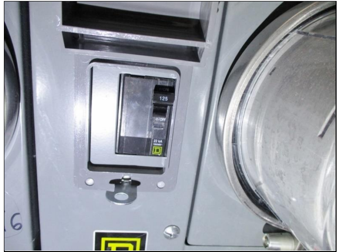
62. Observed 125-amp circuit breaker for residential units in Main building
