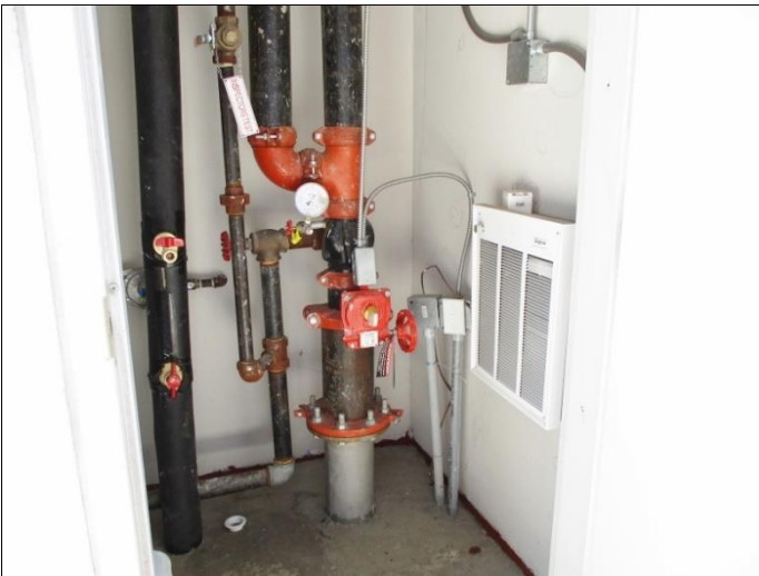
81. Townhome sprinkler riser in exterior-accessed room
