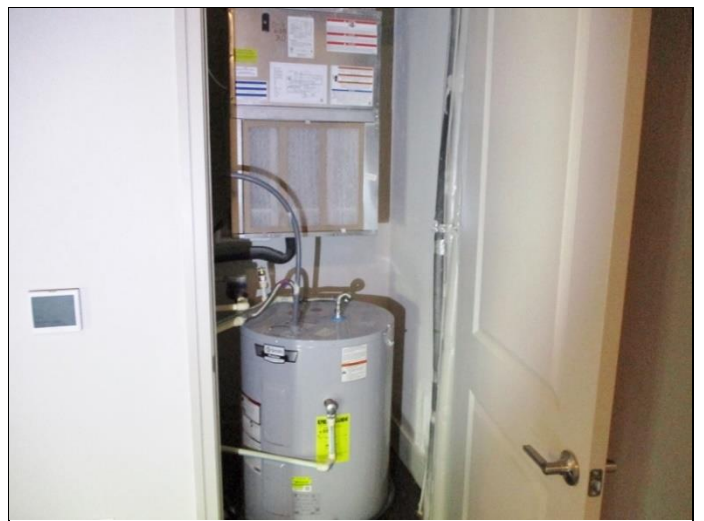
102. Main building tenant interior – HVAC fan-coil unit and domestic hot water heater in closet
