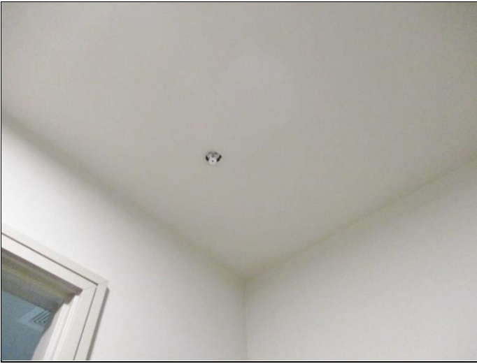
115. Observed missing escutcheon on sprinkler head in closet of Main building unit #825
