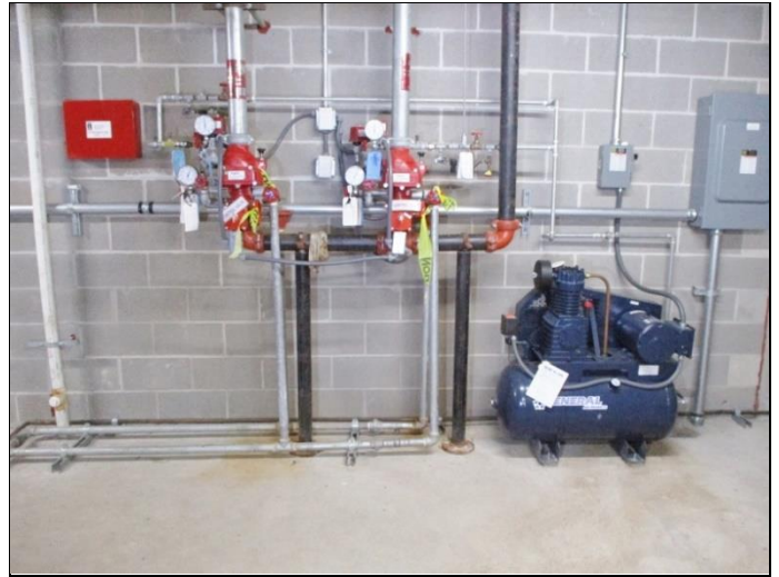
74. Dry-pipe system for parking garage structure
