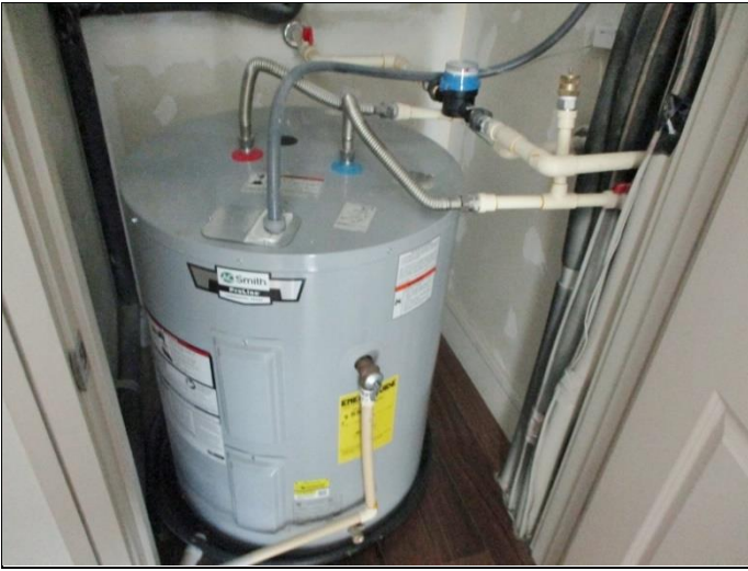
103. Domestic hot water heater with observed water meter
