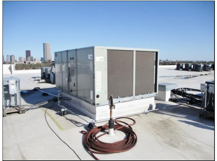
20. Observed packaged rooftop unit for common area corridors
