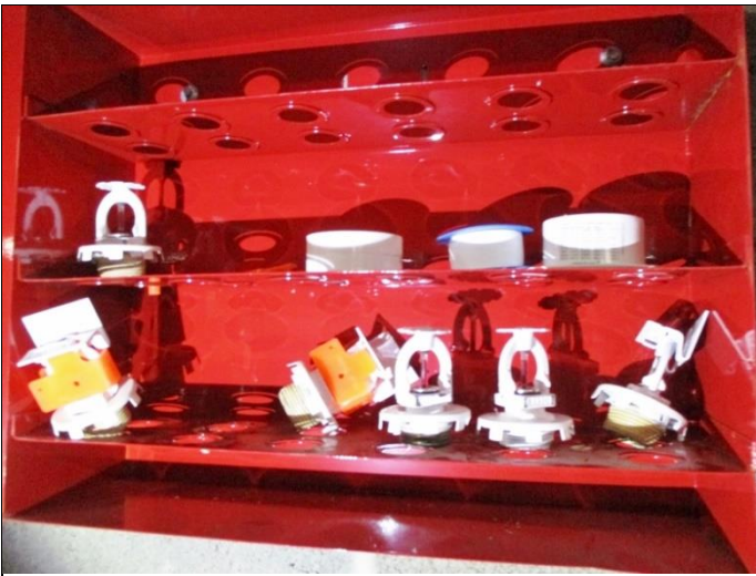
75. Observed sprinkler heads in spare box
