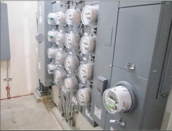
61. Main building upper floor electrical room with tenant electric meters & disconnect circuit breakers
