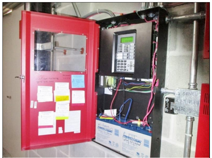
78. Fire alarm control panel
