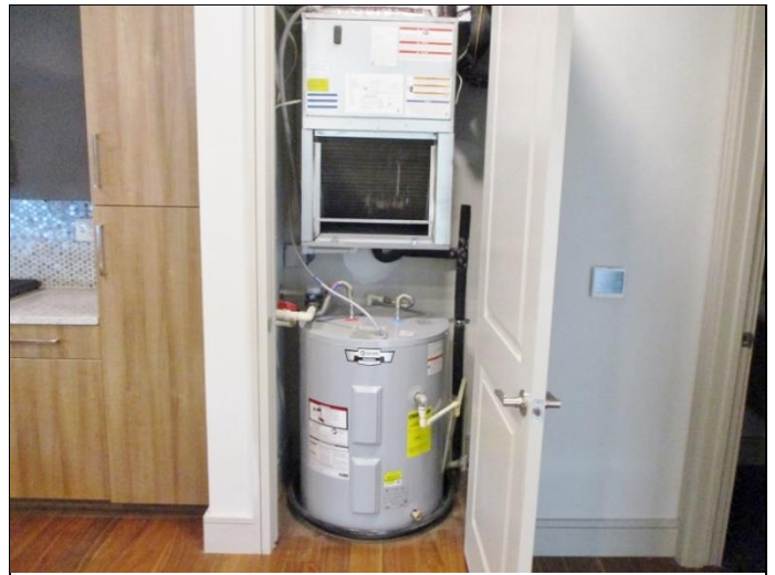
112. Townhome tenant interior – HVAC fan-coil unit and domestic hot water heater in closet
