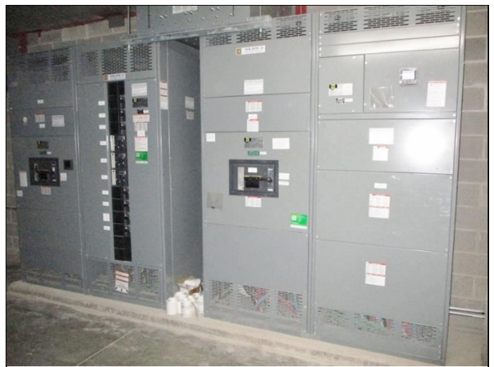
60. Main building electrical service disconnect breaker
