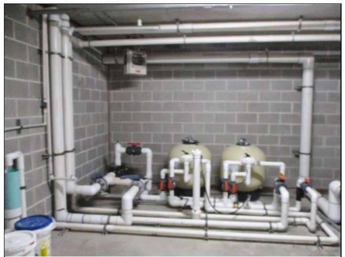
24. Pool equipment in 2nd level parking garage structure equipment space
