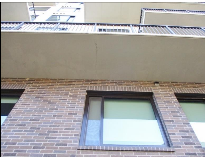
113. Observed cracking on unit #354 balcony on north side of Main building
