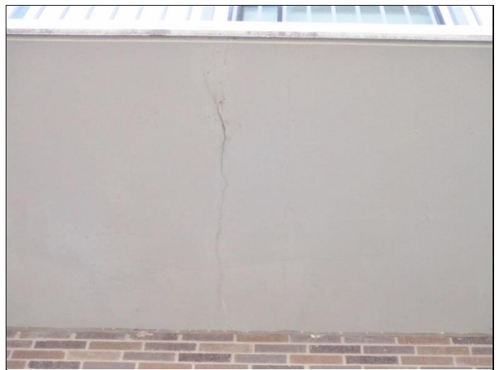
114. Observed cracking on unit #354 balcony on north side of Main building
