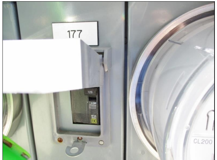
64. Observed 125-amp circuit breaker for residential units in Townhome building
