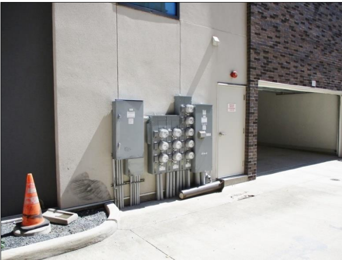
63. Townhome building main electric meters and disconnect circuit breakers
