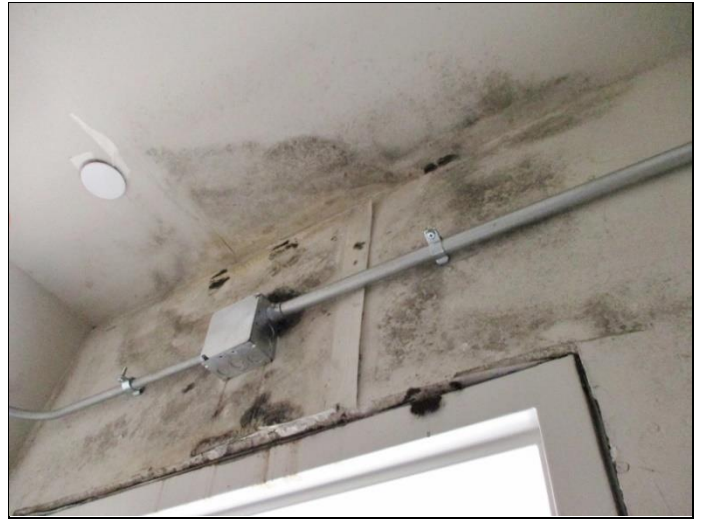
80. Observed suspect microbial growth in Townhome unit #170-174 sprinkler riser room
