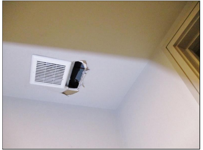
116. Observed hole in gypsum board ceiling requiring repair
